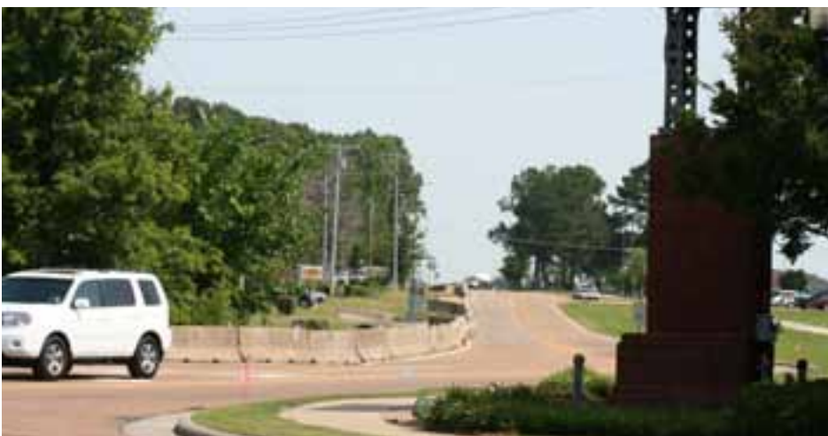
Sunnybrook Road will be realigned during the Phase 1 portion of the project, moving its entrance onto Jackson Street from its current location.
