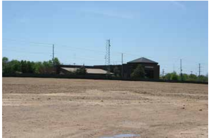
The south half of the City Center project site has been cleared of concrete above and below ground. Plans for the site include a City Hall, a Performing Arts Center, a new Library and a private development area.
