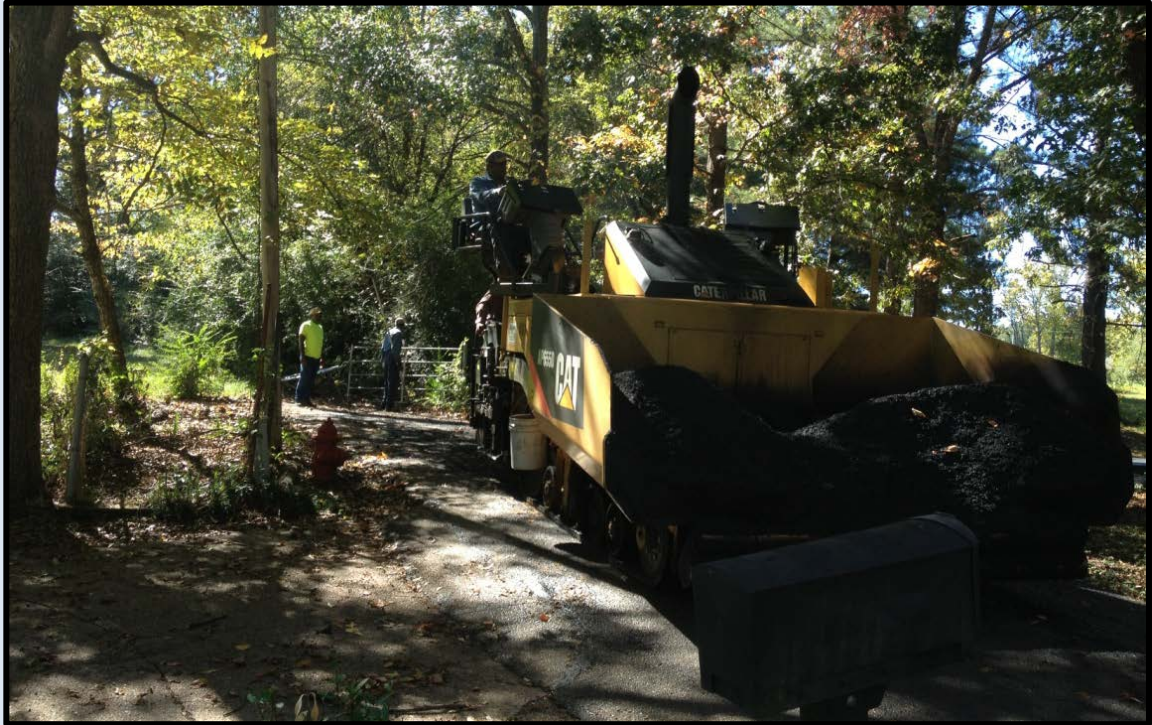
Richmond Grove Milling and Asphalt Overlay
