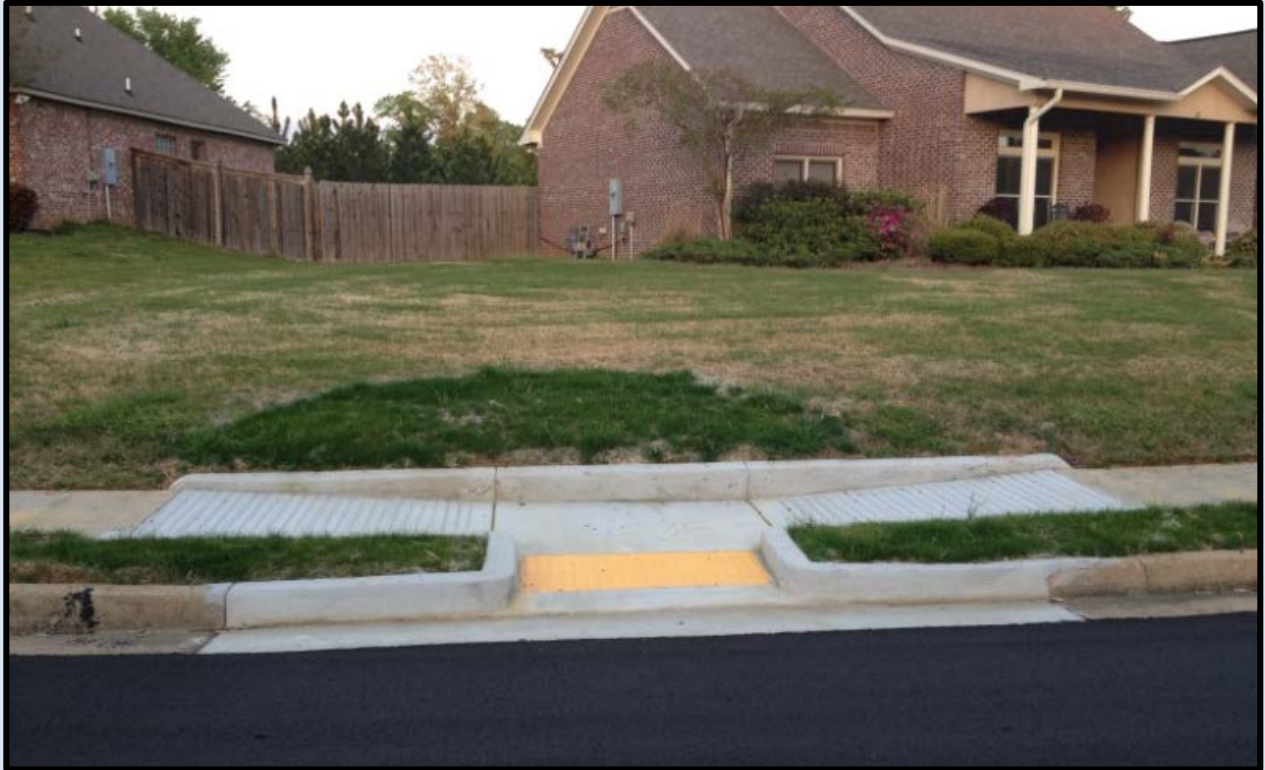
ADA Curb Ramps in Old Agency Village
