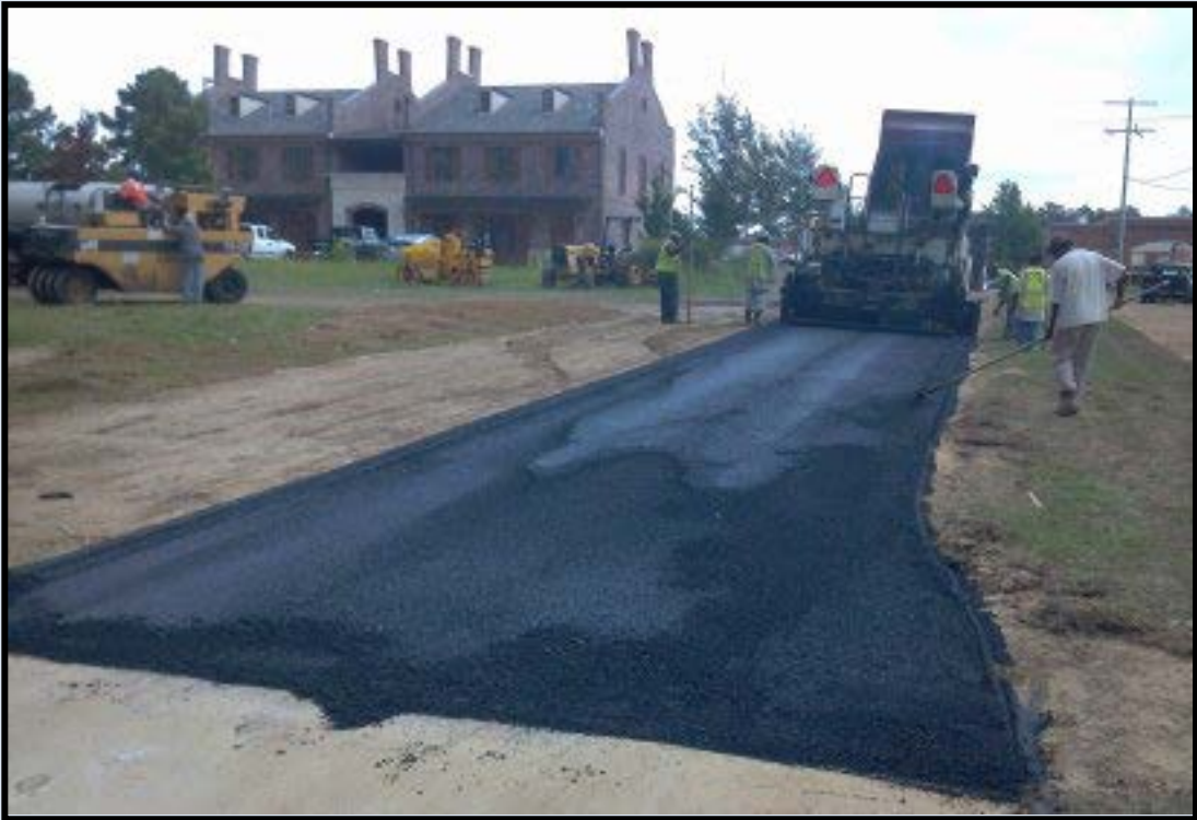
Evergreen Street Asphalt Full Depth Reclamation
