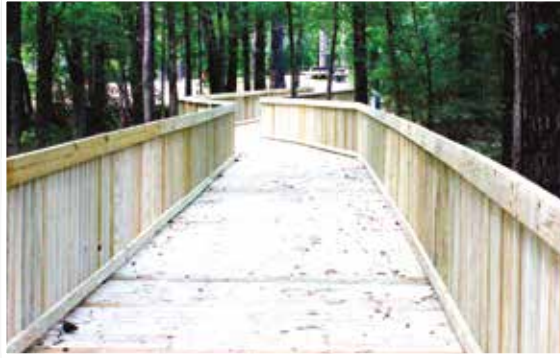
This boardwalk was completed over the summer to connect the Mississippi Craft Center to the Natchez Trace Parkway, making the center directly accessible to the millions of travelers on the Trace.
