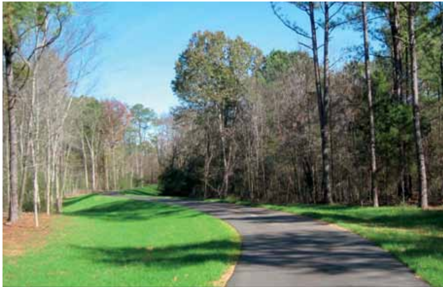
The grand opening of the multiuse trail segment between Old Canton Road and the Reservoir Overlook was celebrated in January, 2011.
